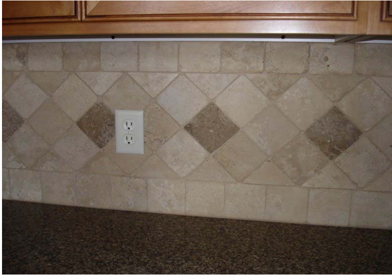
Kitchen backsplash in Mocha Travertine (field) with accents (only) of Beige Travertine
